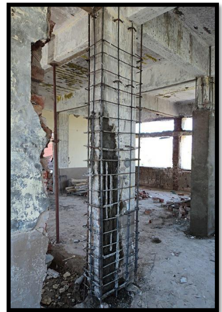
Figure 129 Repair and rehabilitation of Column
